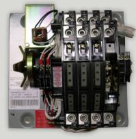
Photo left details 4-pole Transfer Switch used for switching the neutral
